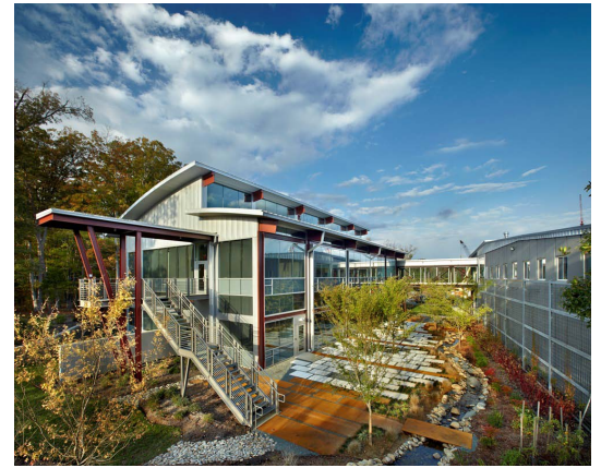
ABOVE: 2012 Engineering Excellence Awards "Grand Conceptor" winner, Stewart Engineering's "Buckner Companies Home Office."
